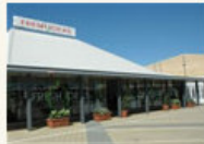
The Fresh Ideas Centre from the outside.
